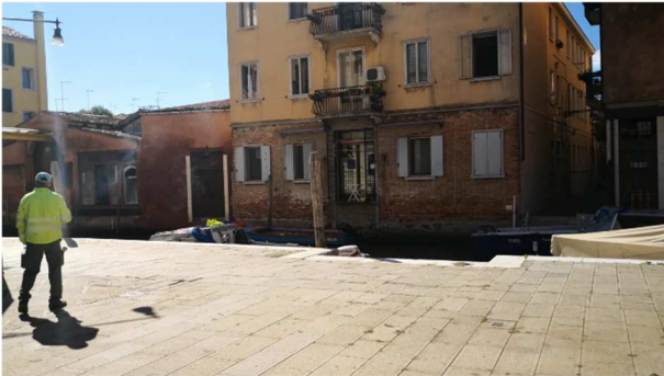
Area vasche interrate
