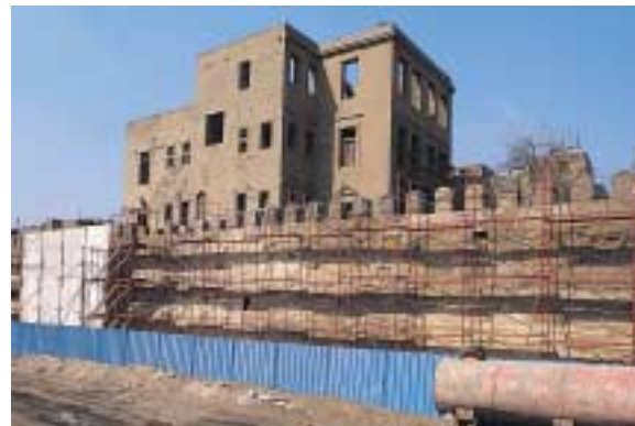
Above: Darb Shoughlan school facility under rehabilitation.
